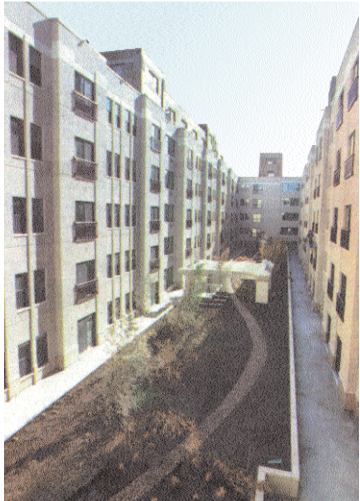
The Left Bank apartments' large courtyard was created by removing the middle of the building. The amount of concrete taken away was enough to form 15 miles of sidewalk. On the left, developer Carl Dranoff talks with Charles Jefferson, the construction director, in the courtyard
