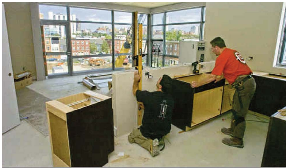
Kitchen cabinetry goes into one of the units at 777. The apartments are aimed at younger professionals and newly arrived executives, both groups that are deferring homeownership.
